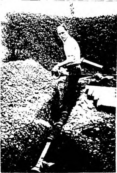
Ted Tapley laying drain
