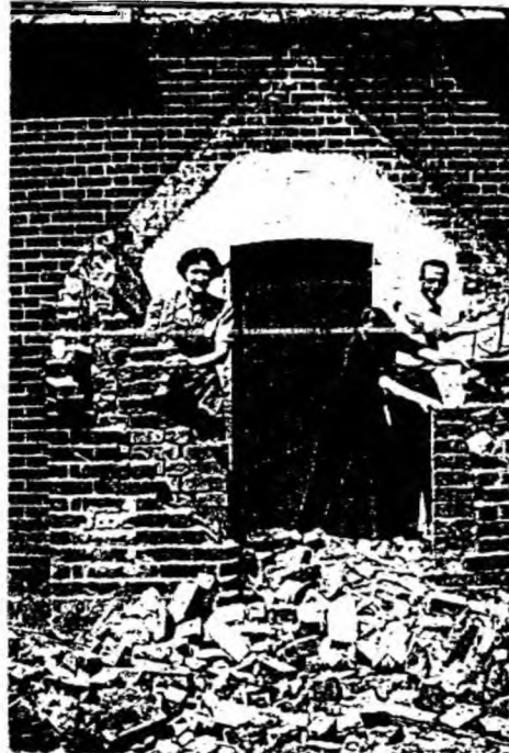
Demolition of porch
